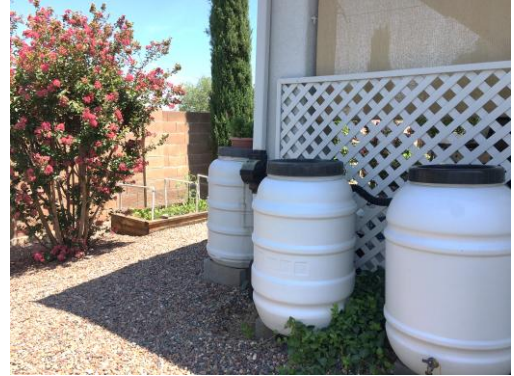
Fig 1 —Three 50-gallon rainbarrels (painted used food drums) supply water for the small garden behind.
